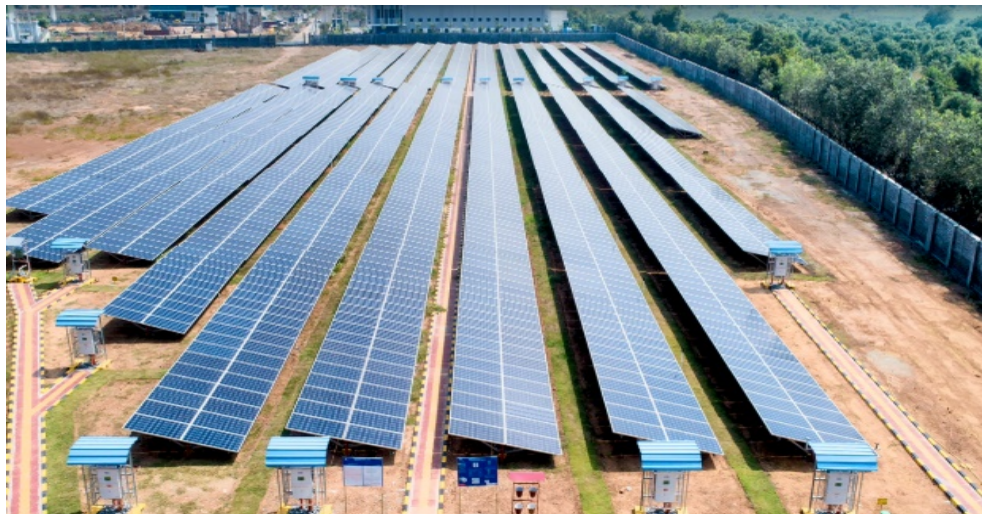
Solar & Wind Installations across plants
